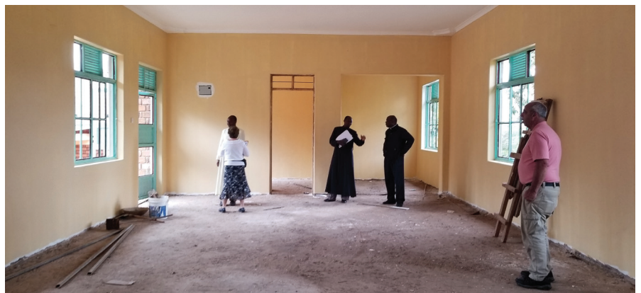
Boys' Dormitory - assessing progress of construction during our Mission trip.
